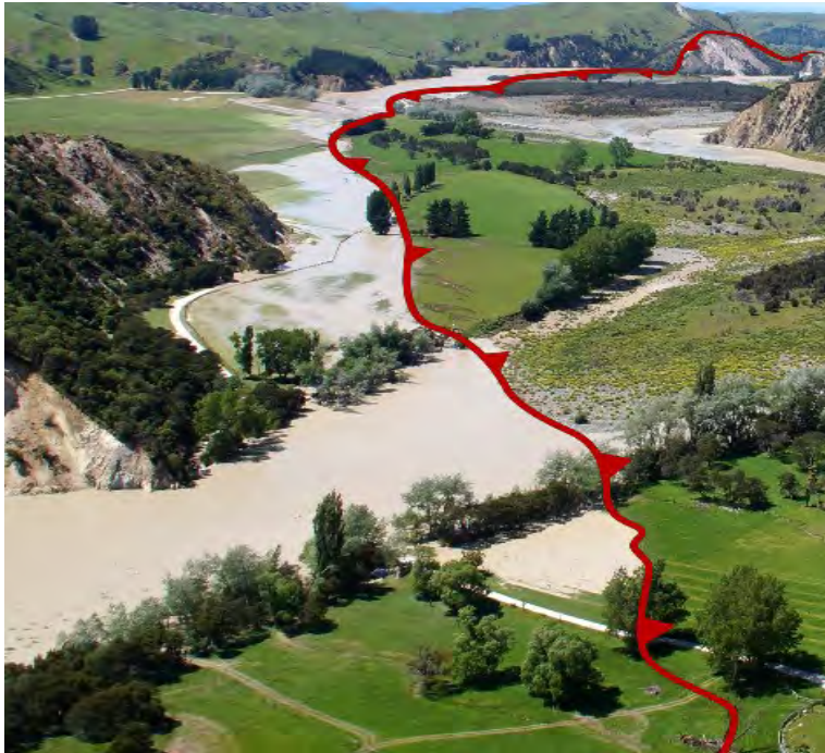
Oblique aerial photo of Clarence River avulsion
